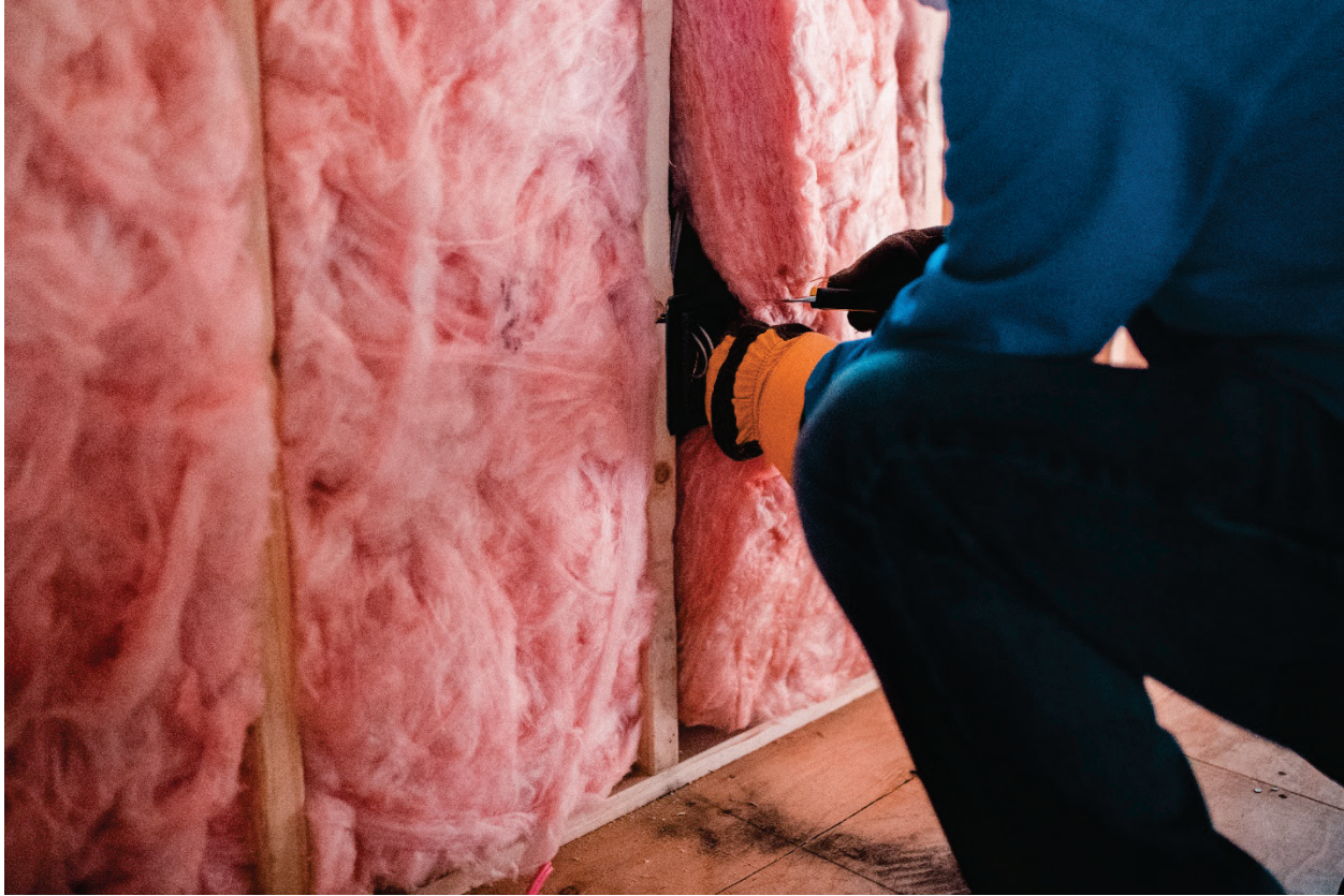
Figure 12. Fiberglass insulation being installed in a residential building.
